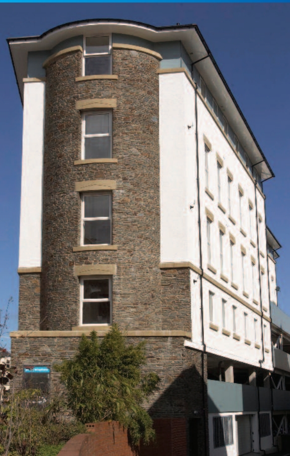
Hanover House Phase 2 - August 2011 providing 12 public sector flats complementing the 15 flats constructed previously in Phase 1
