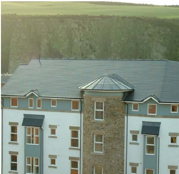
New Housing at Hanover House
